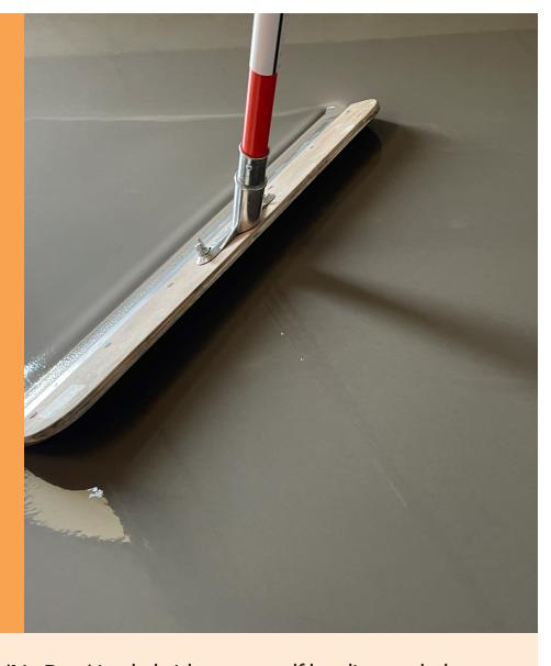
**SKIMFLOW® NP** (No Prep) is a hybrid cement self-leveling underlayment designed for time sensitive projects, where compromised substrates make shrinkage undesirable. **SKIMFLOW® NP** offers no-shrink, noprofile technology to fast-track jobs, without sacrificing performance.
